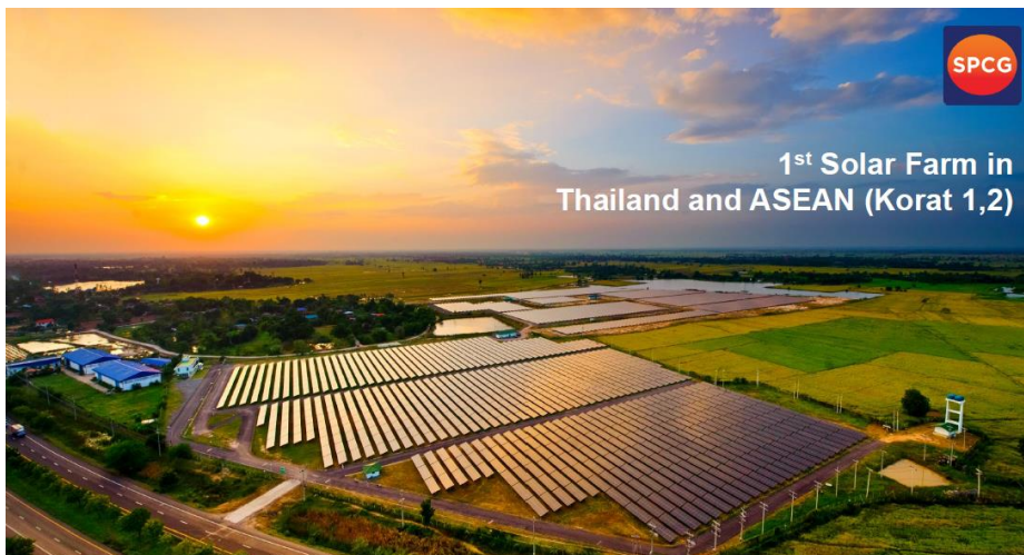
Figure 1: SPCG solar farm
