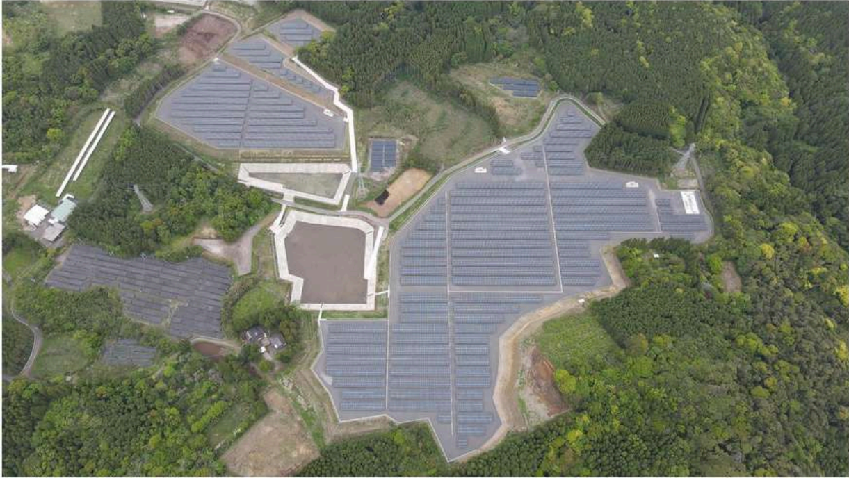
Kagoshima Ohura Mega Solar Project, Kyushu Island, Kanoya City, Kagoshima Prefecture, Japan
