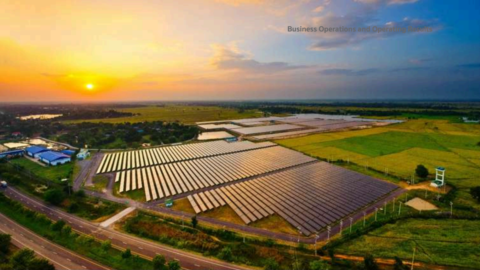
Korat 1 & Korat 2 Solar Farm Projects, Don Chomphu Subdistrict, Non-Sung District, Nakhon Ratchasima Province
