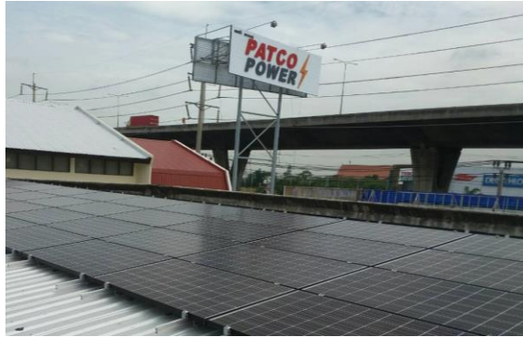
PATCO POWER (53 kWp)
